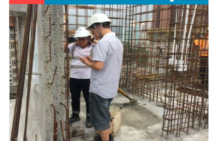
Reading RFID tag after installation
